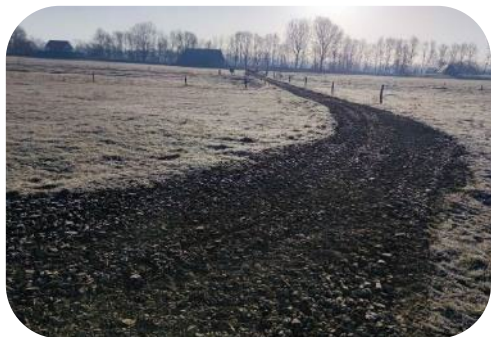
Infrastructure works – road reparations
