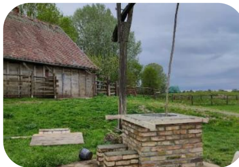
Infrastructure works - building a new well
